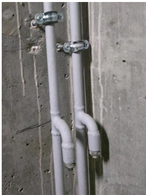
Fig. 3.1. A part of the central heating installation constructed using the black steel pipe welding method (with anti-corrosive coating). Female thread bushes were welded at the raiser bifurcation for further development of the installation in a different technology at the riser branching. (Note: fig. 3.1 – 3.30 - Promotional materials of KAN-therm)
