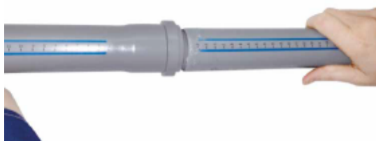
Fig. 3.70. Inserting in the plain end of the pipe into the socket
