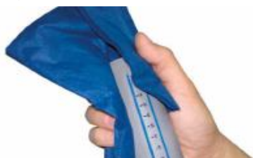
Fig. 3.68. Cleaning the plain end of the PP HTplus pipe
