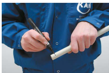
Fig. 3.11. Marking the welding depth on a PP pipe.
