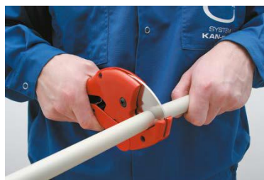
Fig. 3.10. PP pipe cutting.
