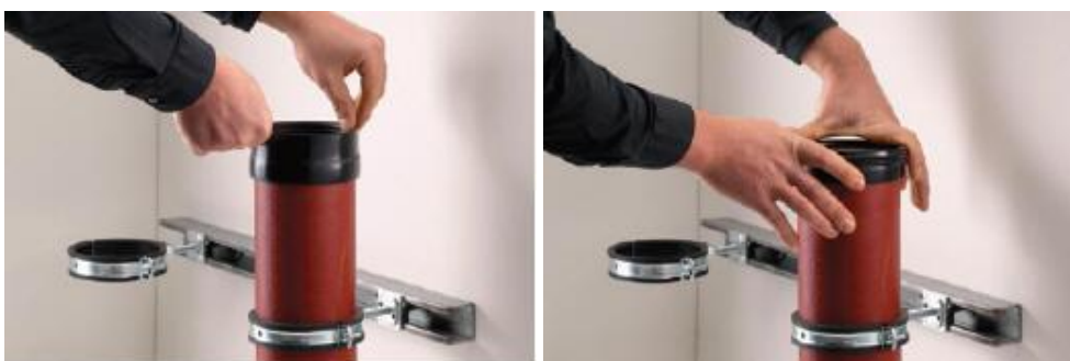
Fig. 3.77. Installation of the rubber bush on the SML pipe produced by KZO (Note: fig. 3.77 – 3.79 - Promotional materials of KZO)
