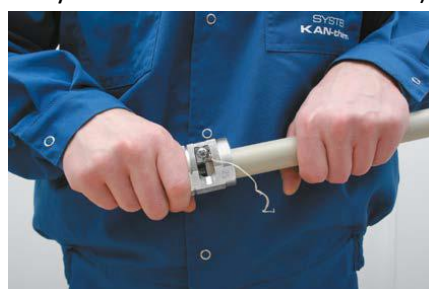
Fig. 3.12. Removal of the aluminium foil from PP pipes.
