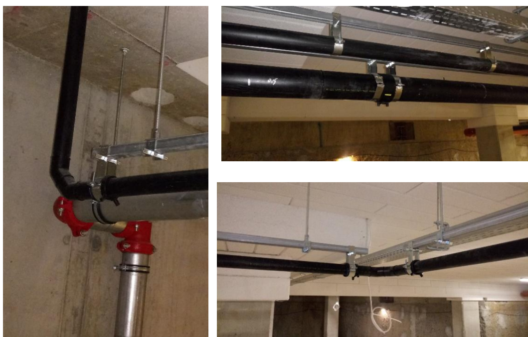
Fig. 3.96. Installation of Pluvia horizontal pipes on system hangers. 2 solutions of fixed points may be observed: by means of 2 grips installed at the electrofusion couplers and by means of a grip and clamp dedicated to fixed points at the change of vertical and horizontal direction of the installation
