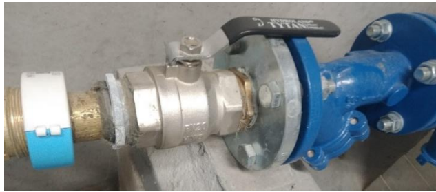
Fig. 3.32. A part of a water supply system connected with threaded joint (on the left) and a flanged one
