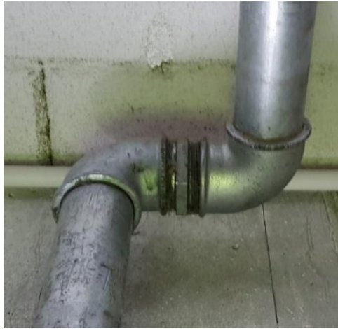
Fig. 3.31. A part of a water supply system consisting of galvanised pipes with threaded joints The valve armature of wider diameters is connected with pipelines by flanged joints.
