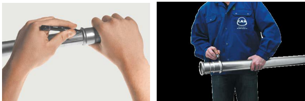
Fig. 3.28. Marking the depth of insertion of a pipe inside a fitting.
