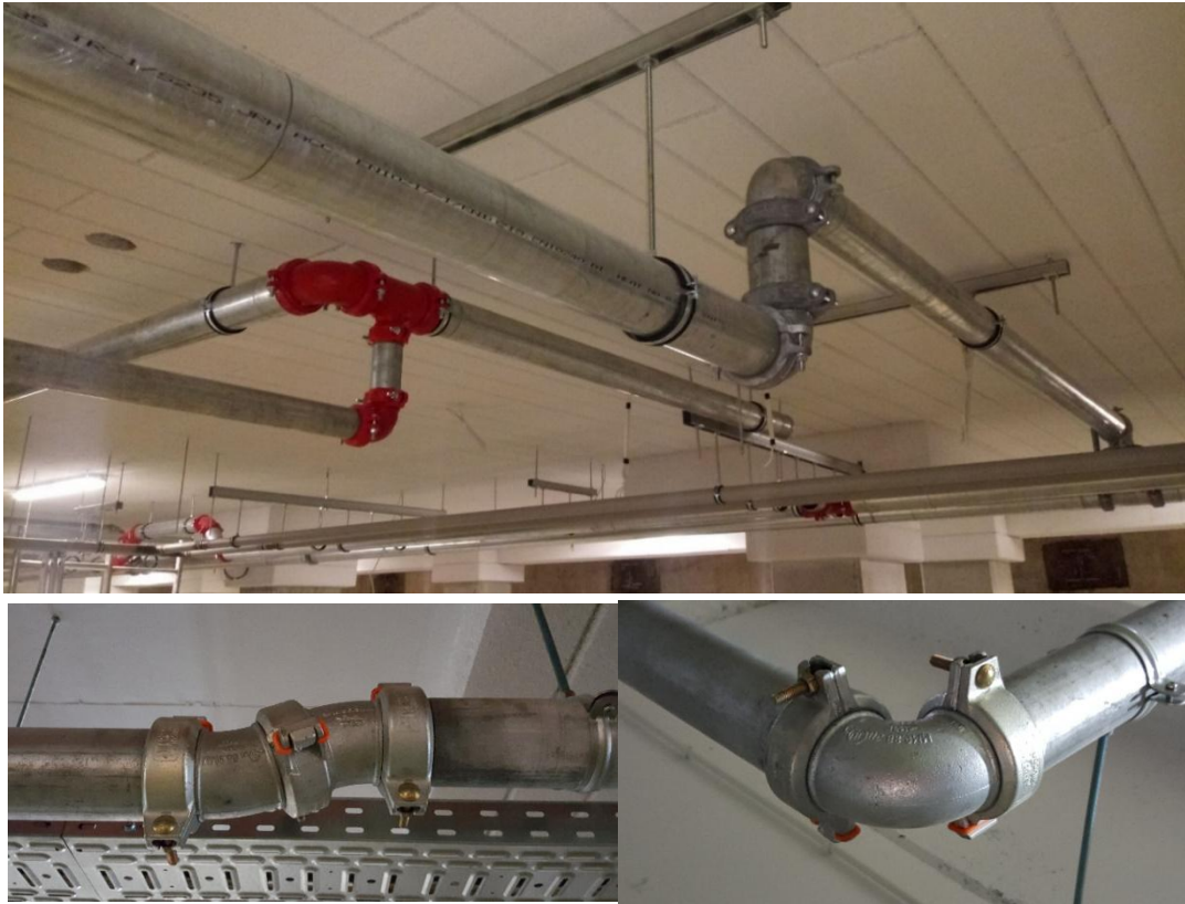
Photo 3.33. Parts of water supply systems consisting of galvanised pipes connected with grooved and threaded joints, part a. (own source)
