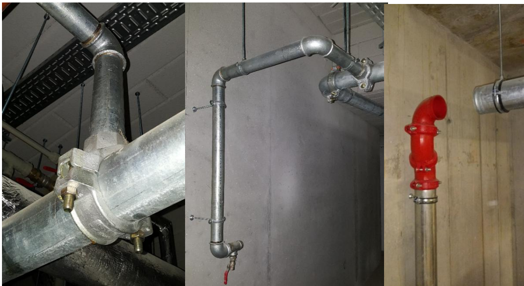
Photo 3.34. Parts of water supply systems consisting of galvanised pipes connected with grooved and threaded joints, part b. (own source)
